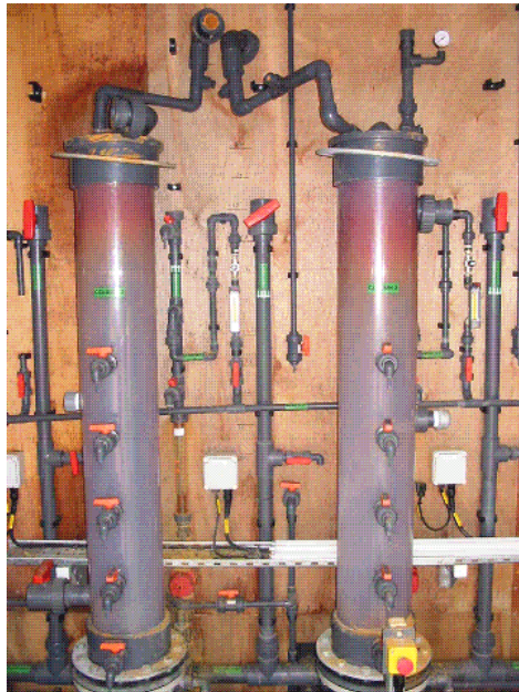
Figure 2.1 AFM and Sand Filter Test Bed Columns – Site J
